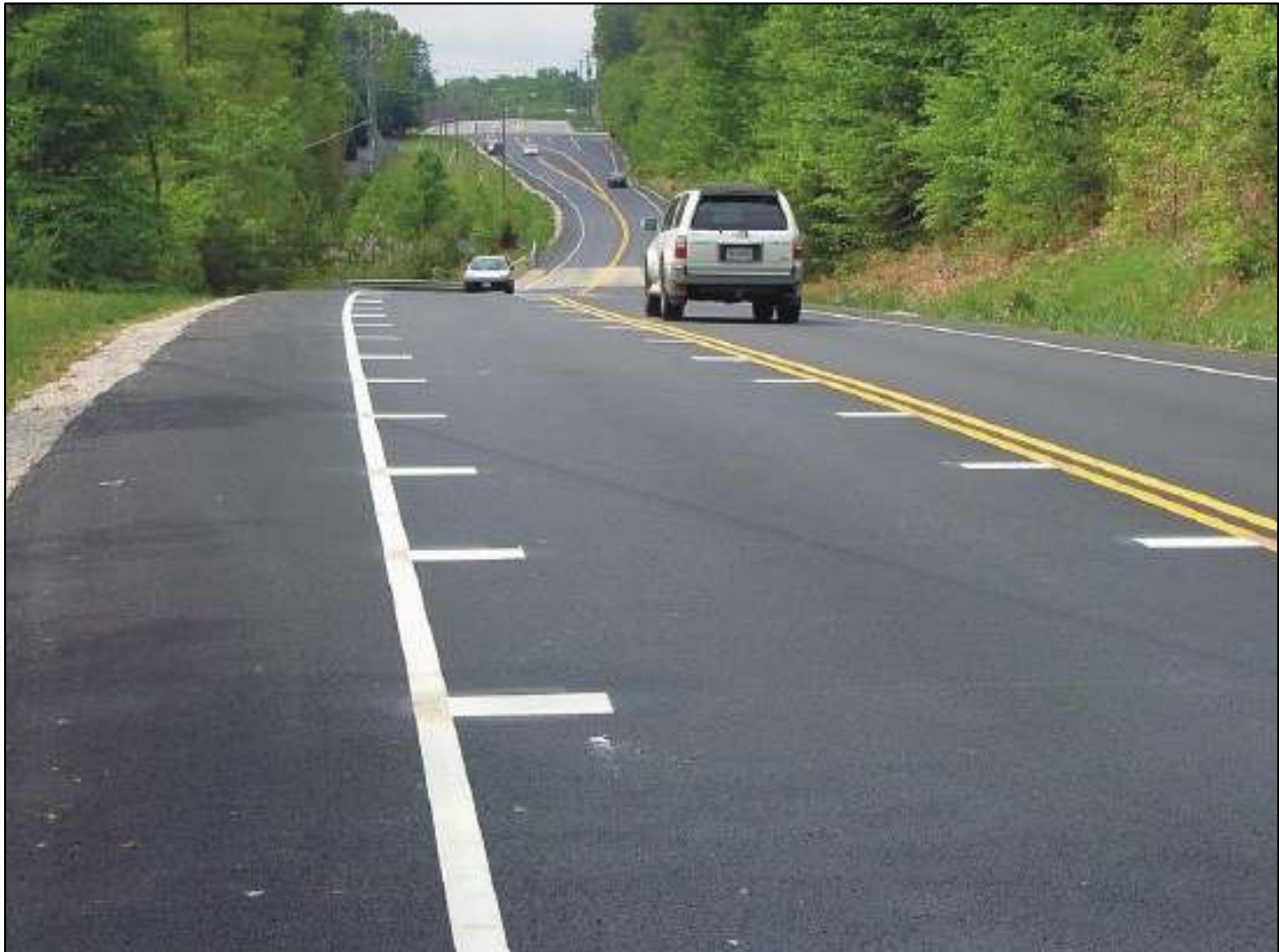
Figure 26: Peripheral Transverse Bars - Image Source: FHWA
