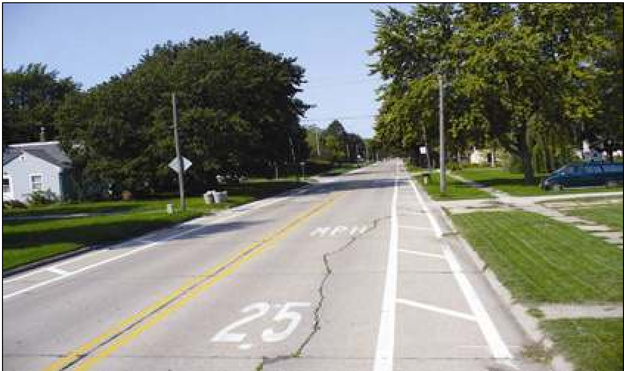
Figure 14: Lane Narrowing - Image Source: FHWA
