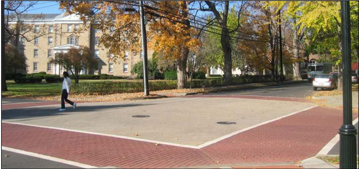
Figure 6: Raised Intersection – Image Source: NACTO Urban Street Design Guide
