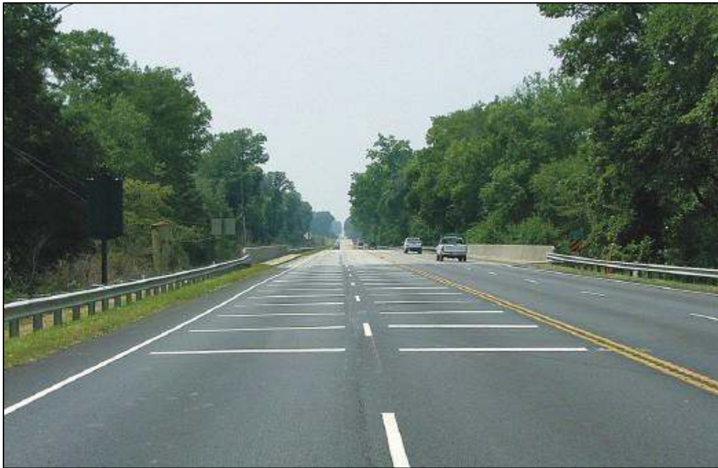
Figure 25: Full-Lane Transverse Bars - Image Source: FHWA
