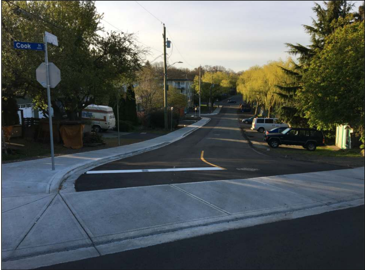
Figure 20: Sidewalk Extension - Image Source: City of Victoria
