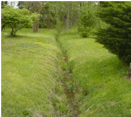
Grass swales infiltrate runoff
